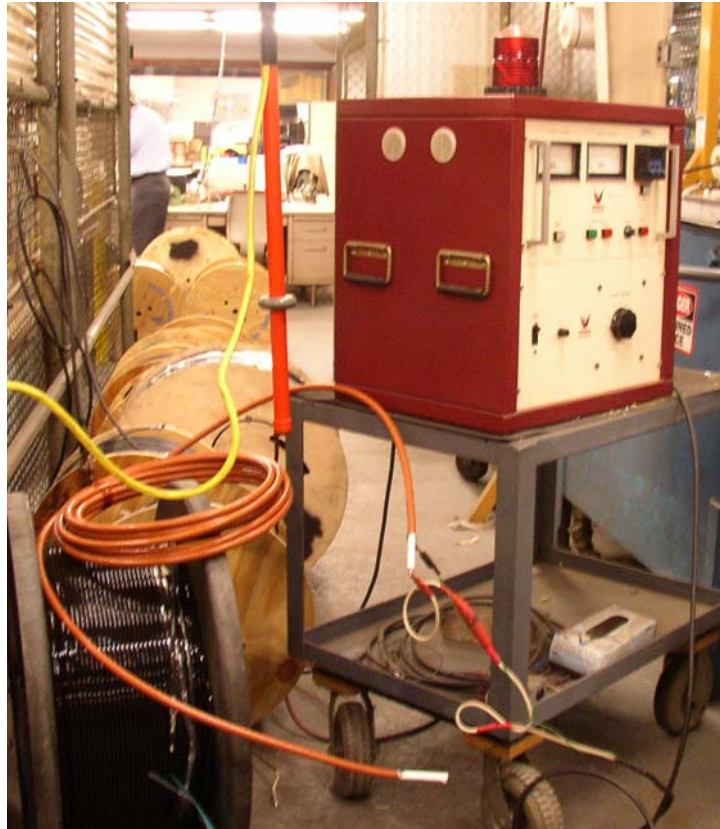
Figure 17 – Voltage Proof Dry Setup
